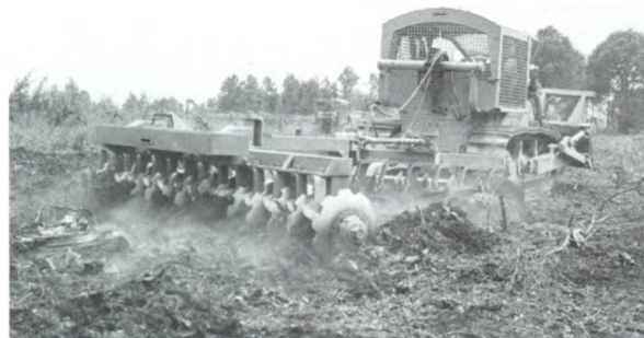
Disking action of the offset disk gangs.
