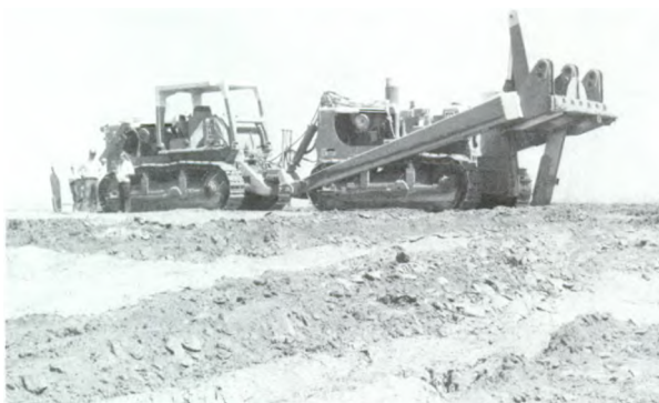
Large ripper for deep penetration.
