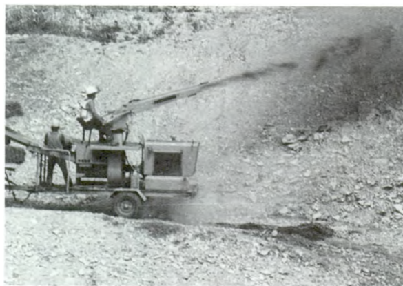
Power mulcher treating a steep slope.
