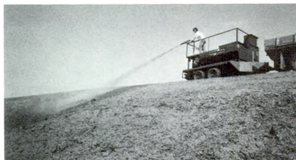
Trailer-mounted hydraulic seeder-mulcher treating a slope.
